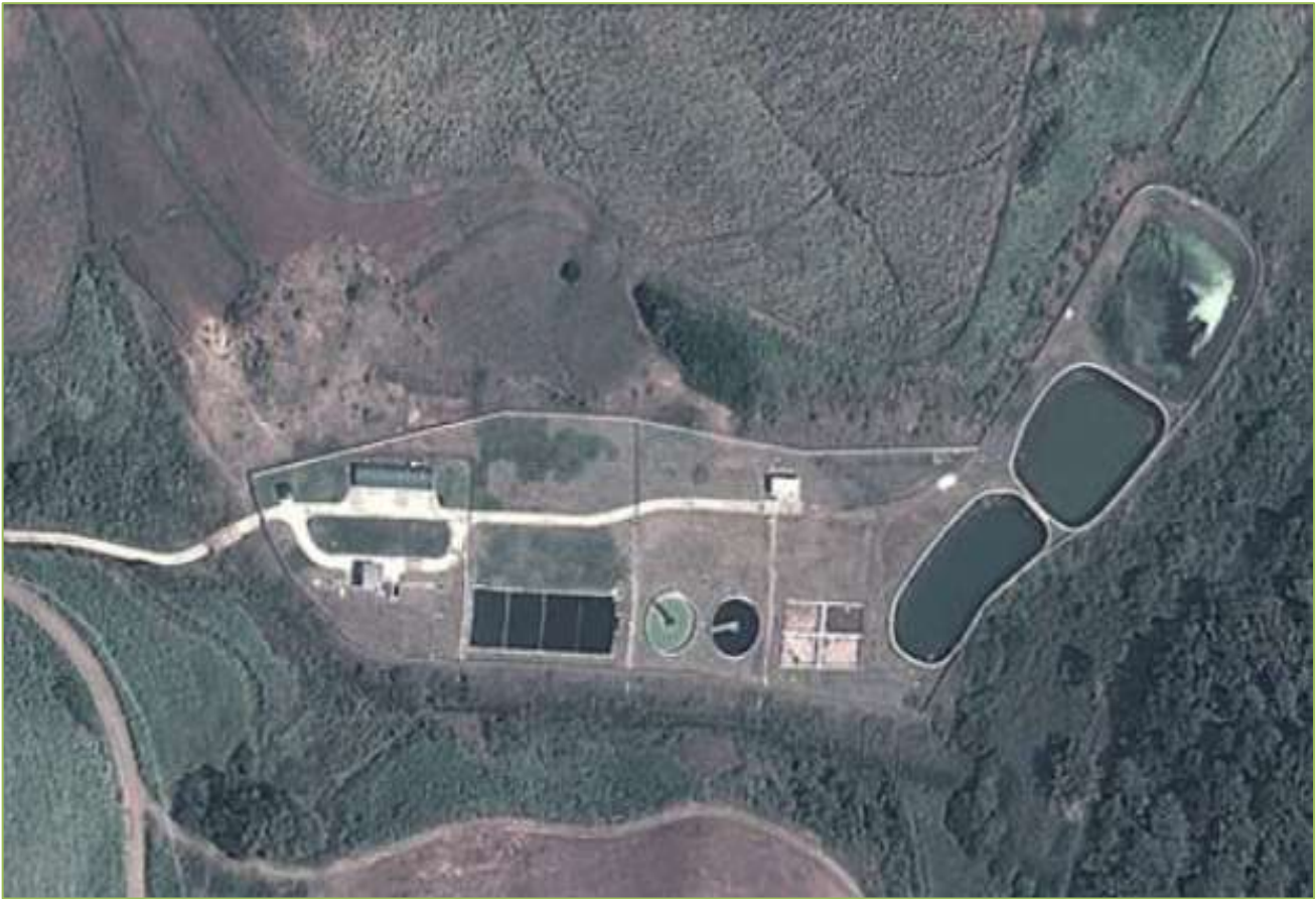
Figure 4-11: The existing Sheffield WWTW
