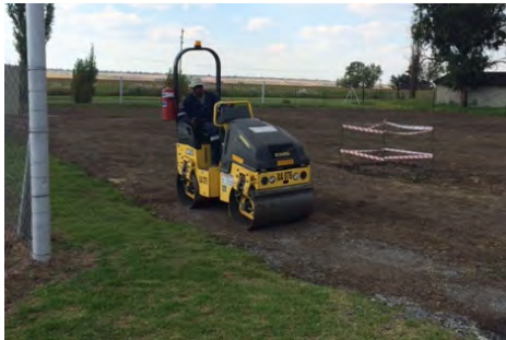
Figure 2: Composting pad preparation
