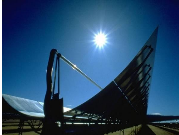
Figure 10: Photo of a trough system 4
