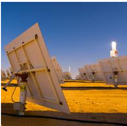
Figure 14: Example of a heliostat 7
