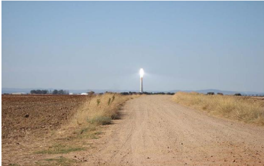
Figure 31 – Central receiver at the Torresol Gem solar Power Plant in Spain
