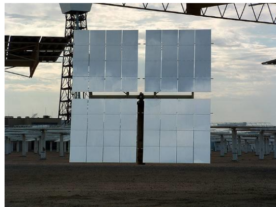
Figure 15: Example of a heliostat 8
