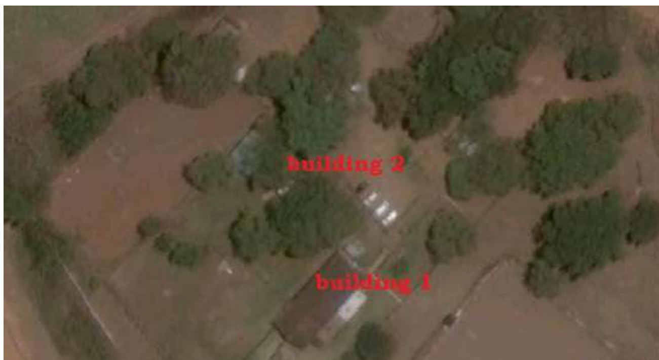
Figure 4-12: Aerial view of site 3
