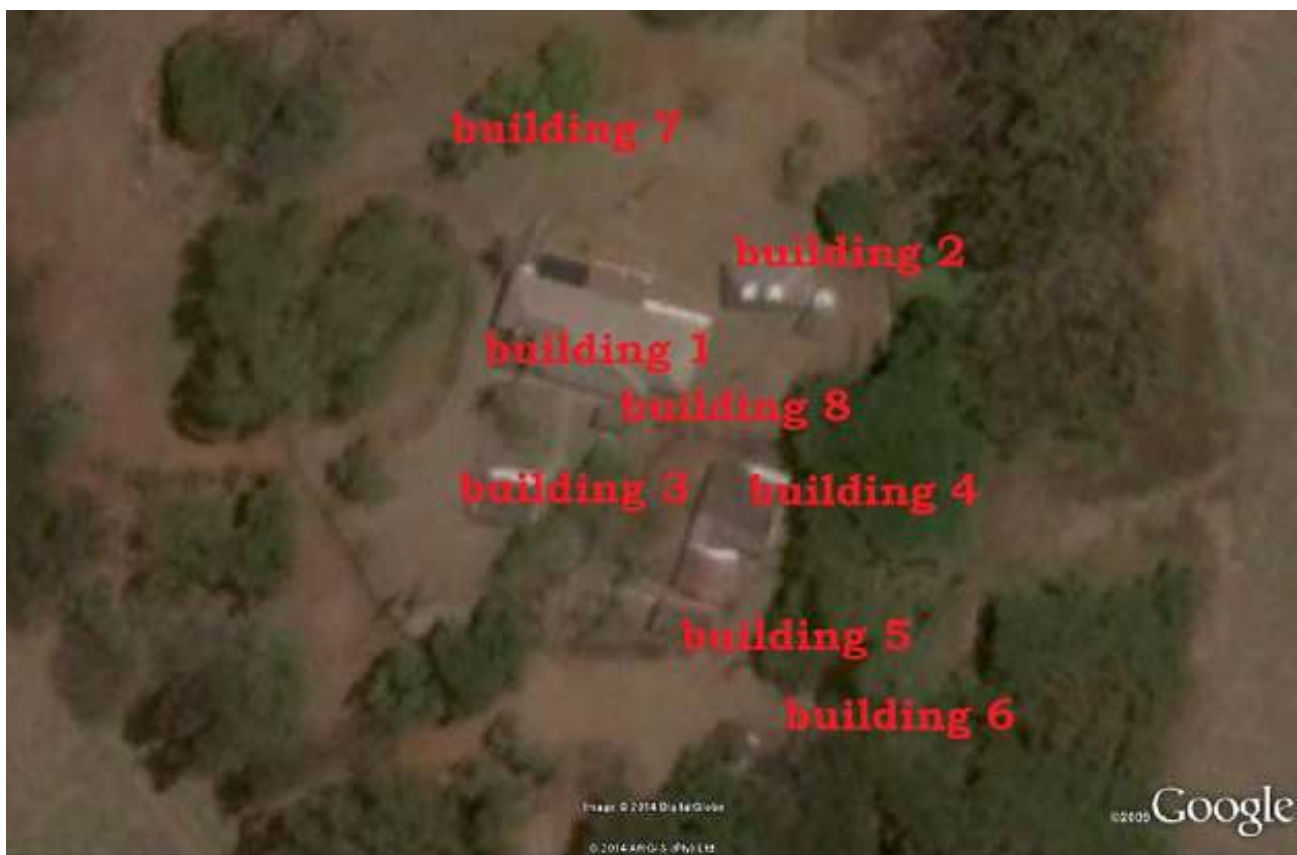
Figure 4-10: Aerial view of site 1
