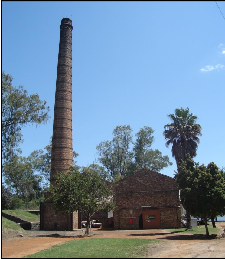
PHOTO 37: WILGERIVIER PUMPSTATION WITH CHIMNEY FOR BIOLERS
