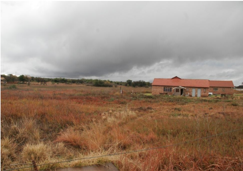
PHOTO 51: A HOUSE BUILT ON AN OLD MINING AREA, NOTE THE WETLAND VEGETATION DUE TO PROLONGED PERIODS OF WATER SATURATION
