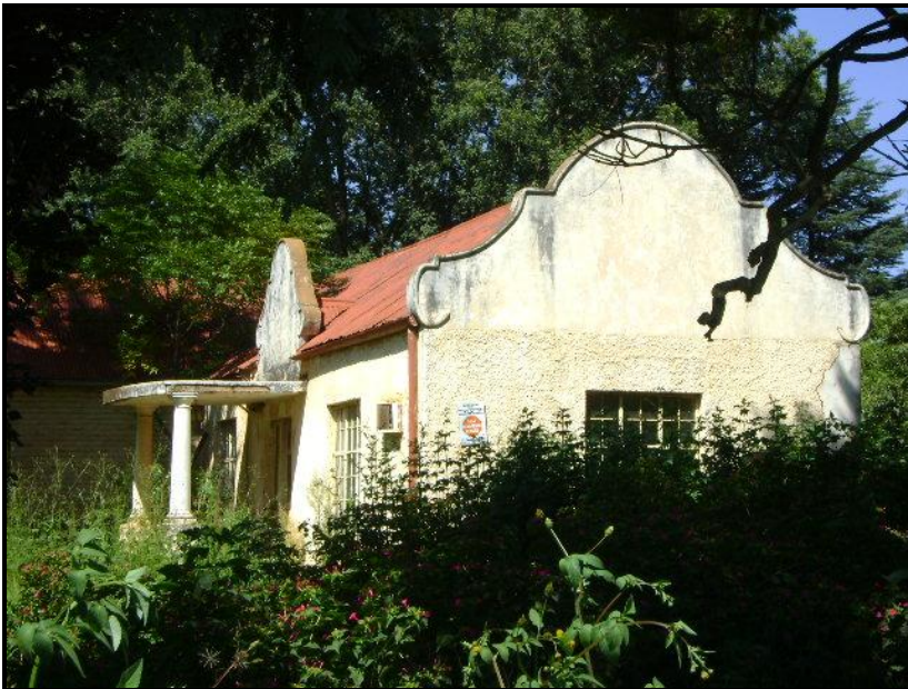
PHOTO 23: 1920'S GABLED FARMHOUSE
