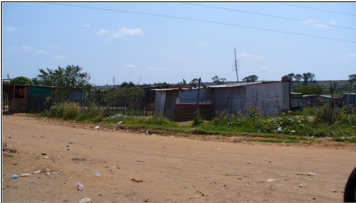
PHOTO 1: INFORMAL HOUSING IN ZITHOBENI
