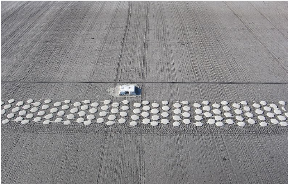
Photo 11.7.6: Raised Thermoplastic Line
