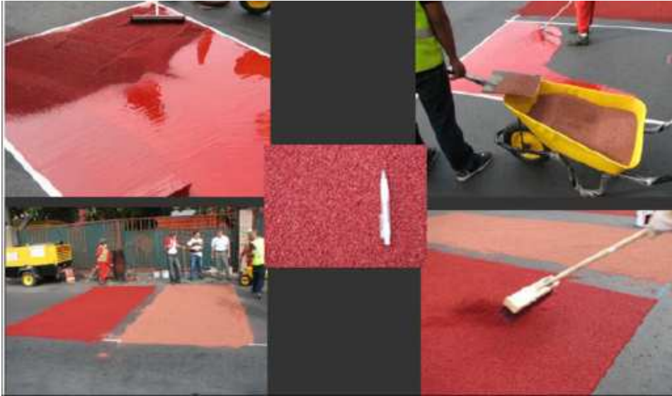
Photo 11.7.7: MyCiti Trial Section of Tyregrip coloured surface application (Photo – SATC 2011 Presentation, “BRT Infrastructure in Cape Town”, HHO)
