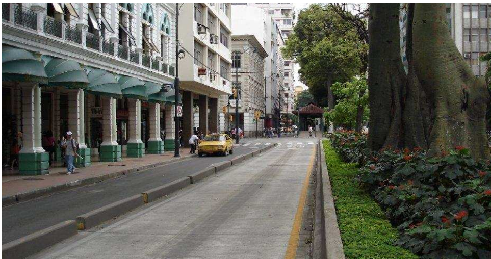
Photo 11.7.1: Barrier Kerb Separator in Guyaquil, Ecuador (Photo – L de Beer, GIBB, 2007)
