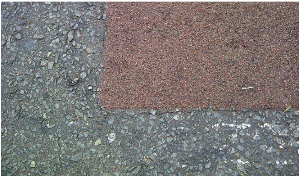
Photo 11.7.8: Tyregrip surface application, Rea Vaya Trial (photographed 3 years after application in 2008) (Photos – L de Beer, GIBB, 2011)
