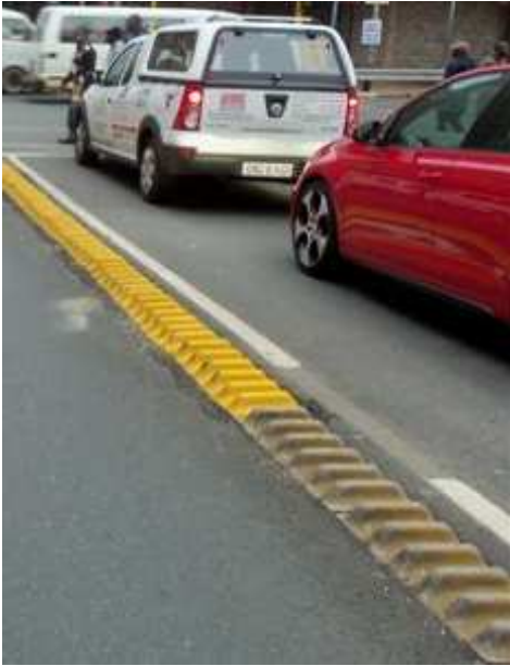
Photo 11.7.4: Concrete Rumble Block, Rea Vaya (newly painted and faded/worn contrast)
