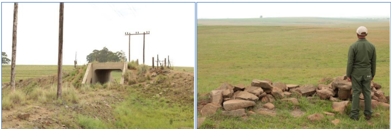
Photograph 18: Old concrete bridge and hunting blinds
